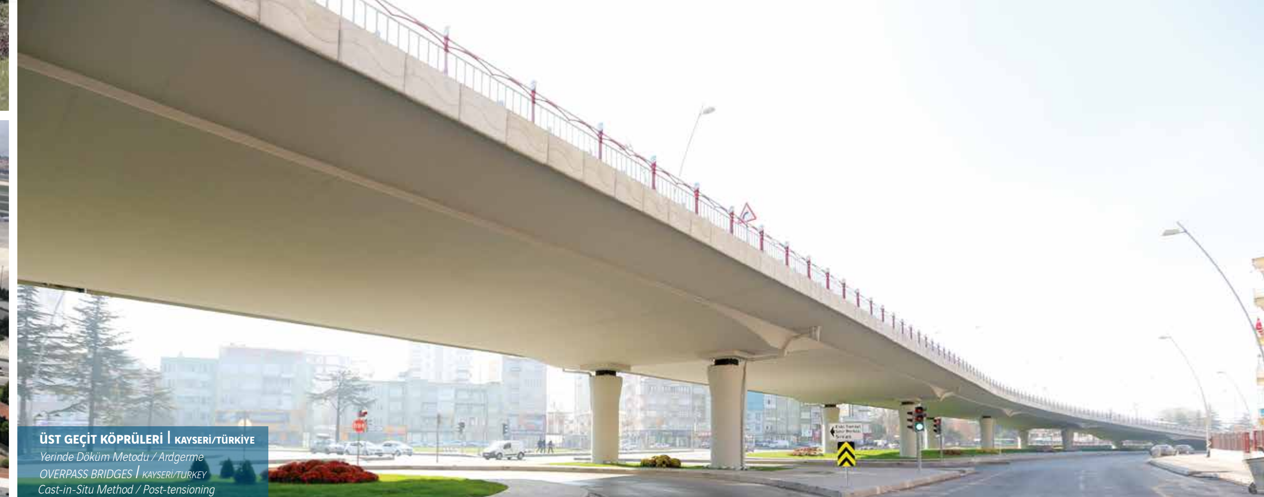
ATATÜRK HAVALİMANI KAVŞAKLARI | İSTANBUL/TÜRKİYE Yerinde Döküm Metodu / Ardgerme ATATÜRK AIRPORT CROSSOVER ROADS | İSTANBUL/TURKEY Cast-in-Situ Method / Post-tensioning
