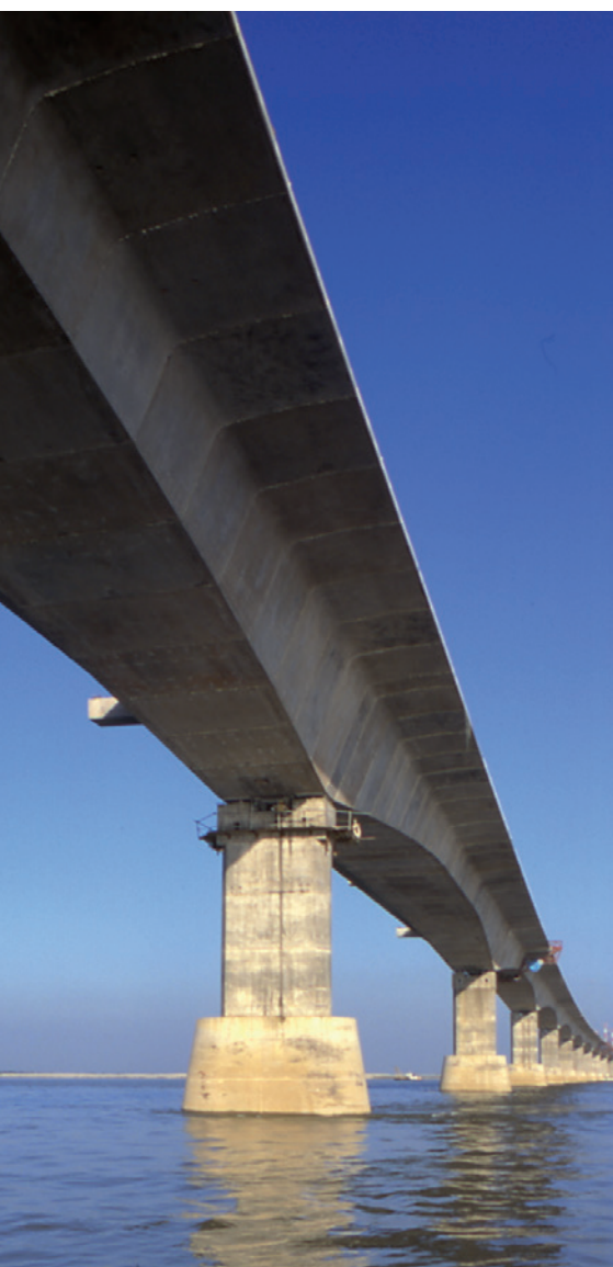
Jamuna Bridge, Bangladesh
