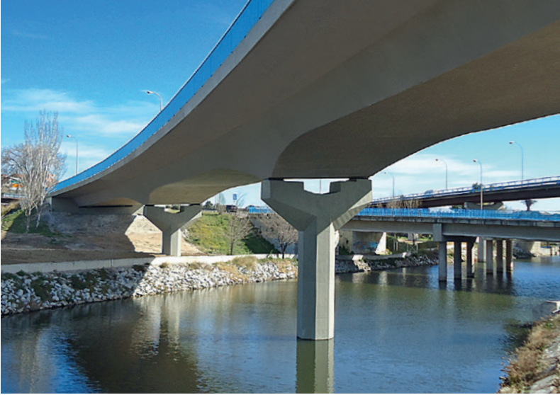
Nudo Sur Bridge on the M-30 Spain
