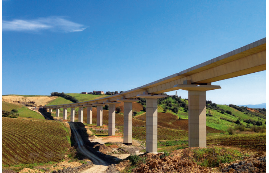
BTZ railway line, Algeria
